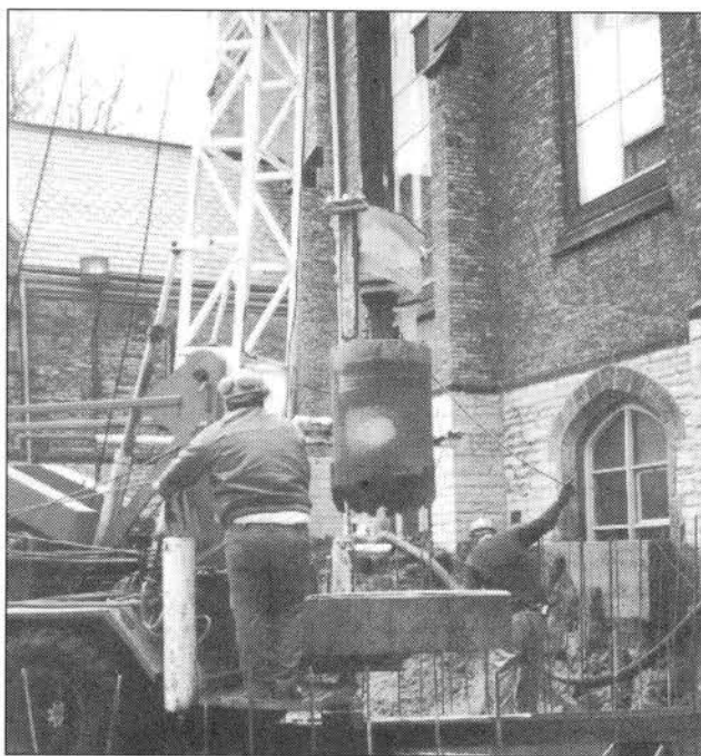
Drilling for oil at FSA.
