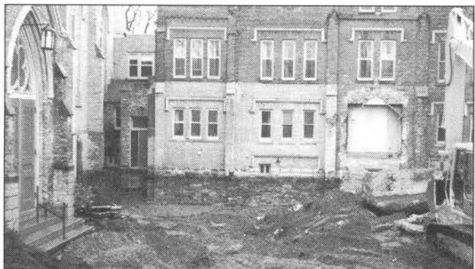
Excavation of the site. April 12, 1994.
