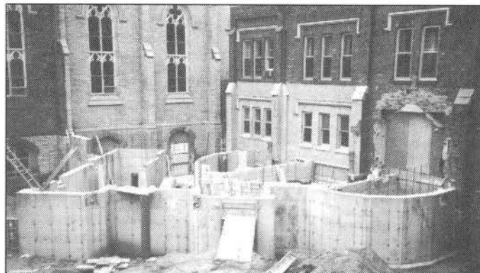
The basement walls are added.
