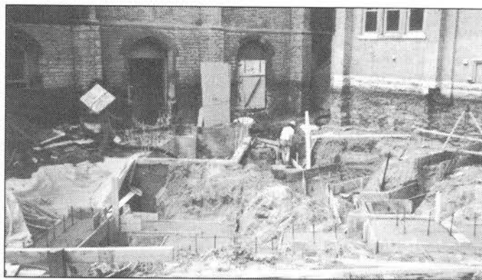
The foundation is poured.
