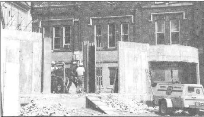
The entrance and main floor walls take shape. July 14, 1994.
