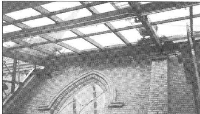
The glass in the atrium is being installed.
